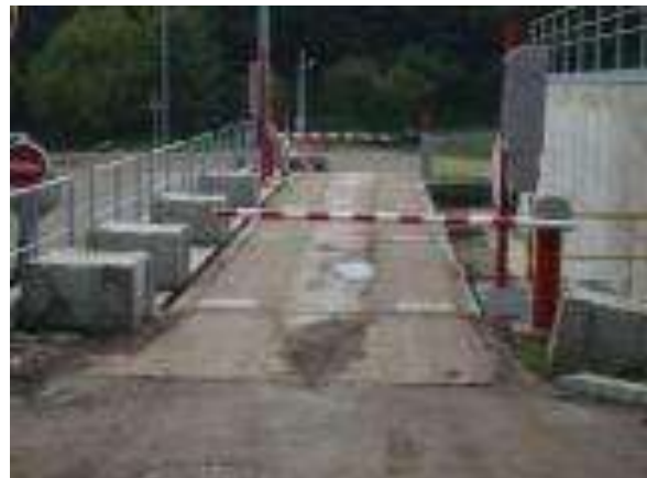
Figure 8.2: Weighbridge at WTS in Rouen, France
