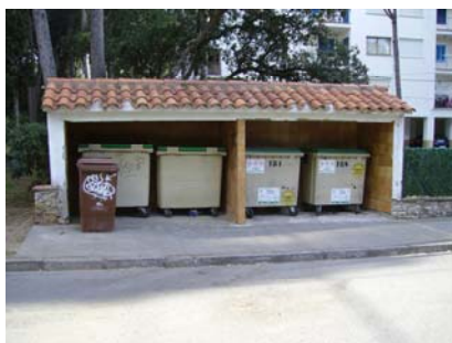
Figure 2- Flat bin store with communal organics and residual waste bins
